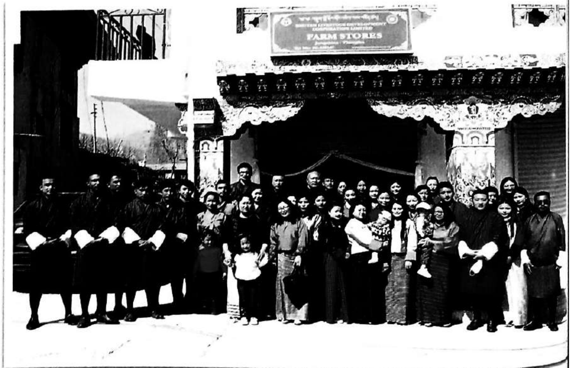
BLDC Outlet, Jungshina, PT House Building, Thimphu
